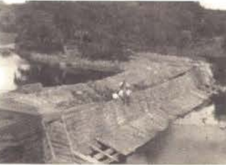
Second construction of dam with railroad ties.
