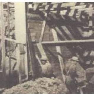
Workers updating raceway which leads to subbasement.
